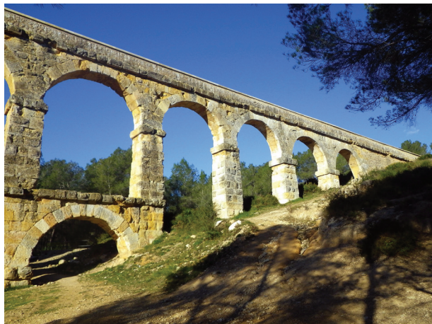
Figure 9.16 —Arched Roman bridge/aqueduct; Roman architects could span deep valleys with arched structures (photo: David E. Graves)
